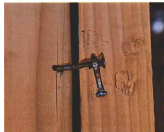
Trimmers are fastened with the help of a single 16d nail connecting the trimmer and the king stud (top left photo). Here the author levers the two members apart slightly while keeping an eye on the level bubble and the gap between the trimmer and the level. The friction of the nail will hold the trimmer and king stud in the correct relationship while the two are clipped together. Clamping a level to the head jamb allows you the freedom to hold a ½-in. thick block along the edge of the side jamb, approximating the wall-sheathing thickness (photo above). A pair of 8d nails that have been bent over to clip the trimmer and the king stud can be seen in the photo at left.
